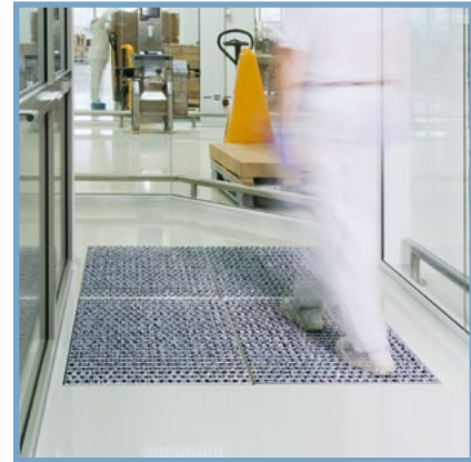
Ebenerdiger Einbau von ProfilGate® GO In-ground installation of ProfilGate® GO
